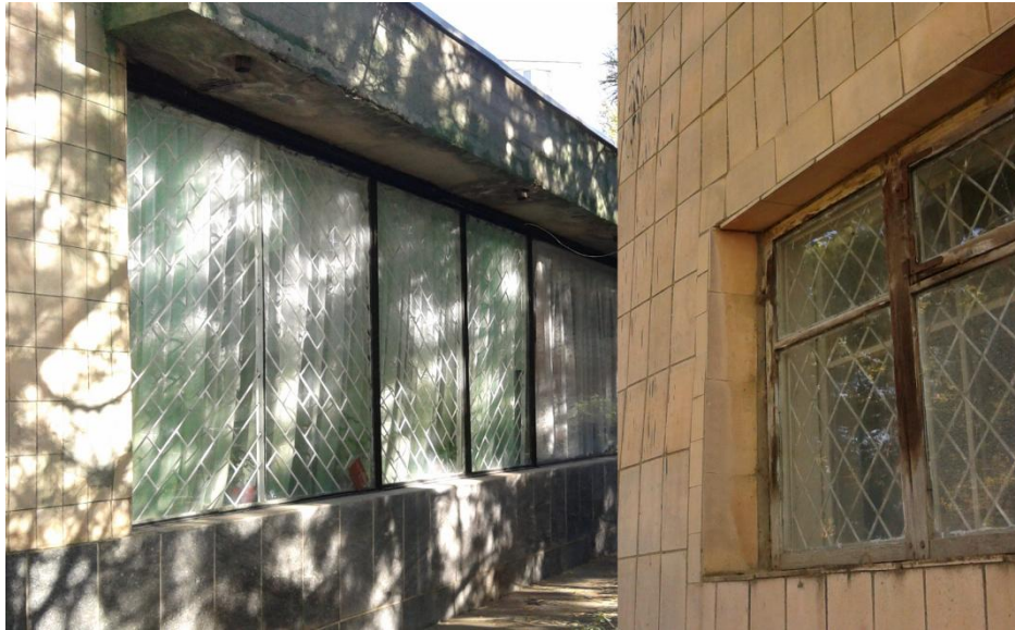
10. figure: Windows with steel or wood frames
