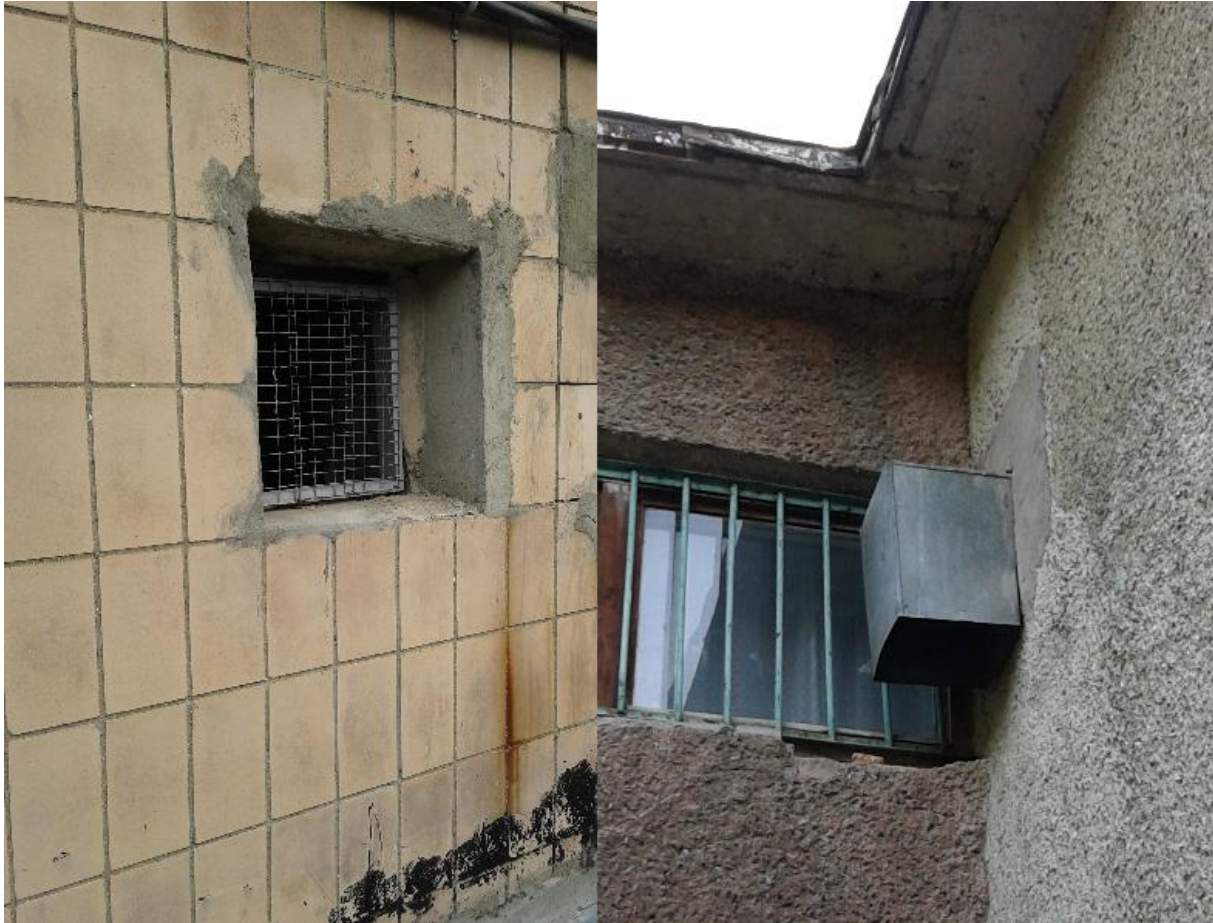
14. figure: Ventillation openings
